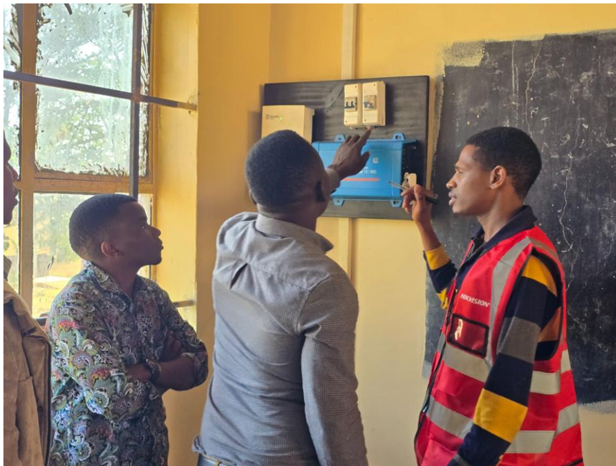
Solar Technician gives teachers instruction of power system during installation.
